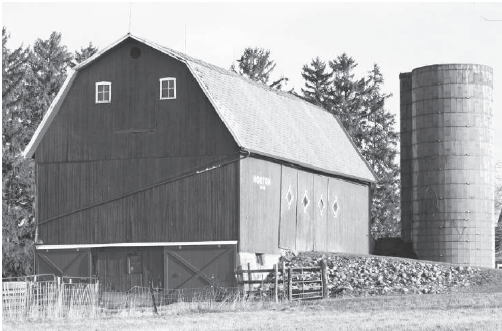
This barn has a gambrel roof and features an area on the ground floor where cows were milked and a second floor where hay and straw were stored. The hay mow was accessible to a horse-drawn wagon and later a tractor-and-wagon via an incline constructed of dirt and rocks.
