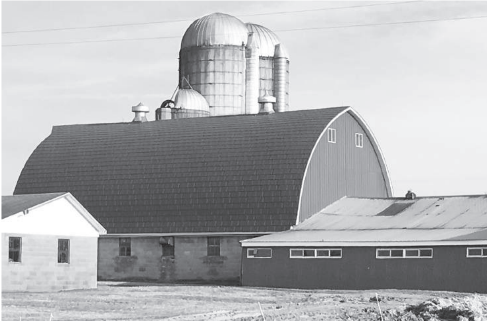
This barn features a gothic style roof and came into vogue in the 1920s.
